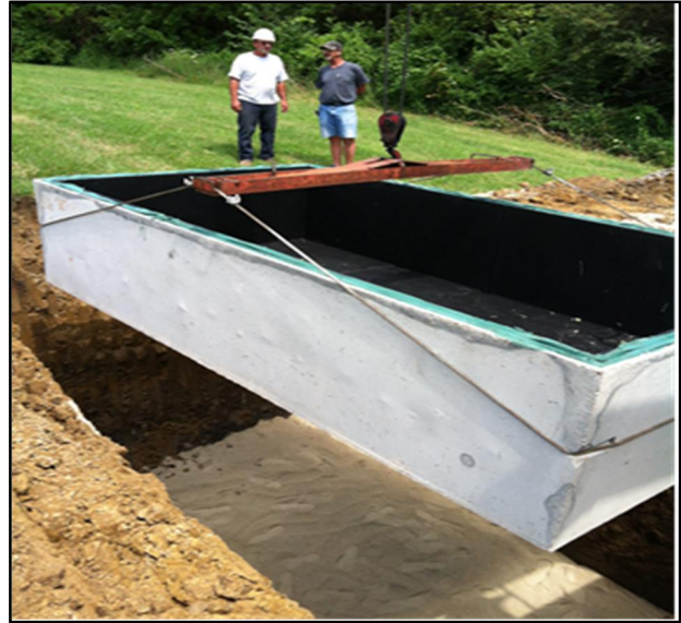
Installing Lift Station Basin at McMahan's Mobile Home Park
